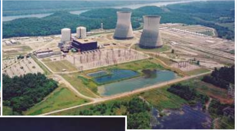
Nuclear Power Plant
